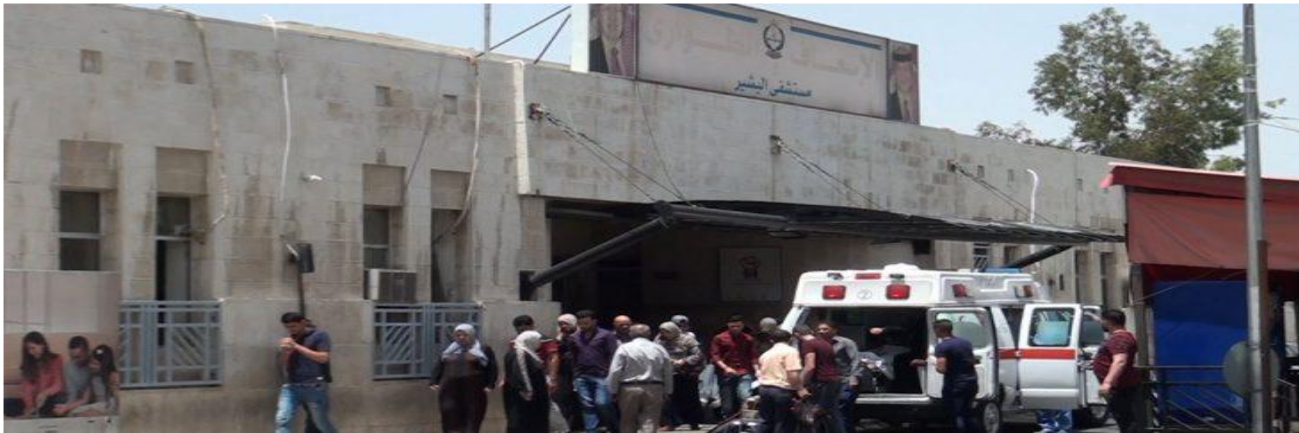
Bashir Hospital – Emergency Bldg.
