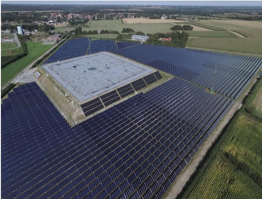
Solar District Heating with Seasonal Storage Pit in Gram - Denmark
