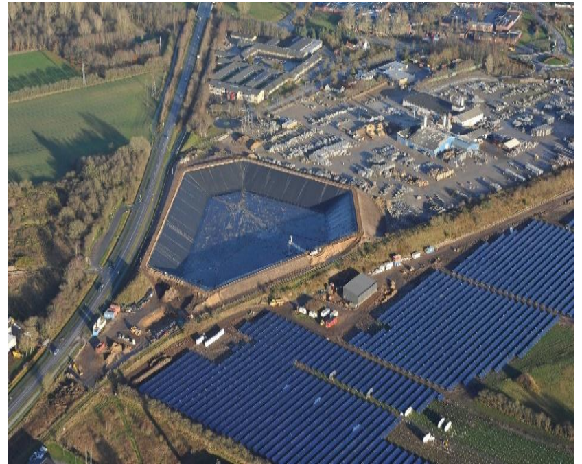
70,000 m 2 Solar District Heating field with Seasonal Storage Pit of 200,000 m 3 in Marstal - Denmark
